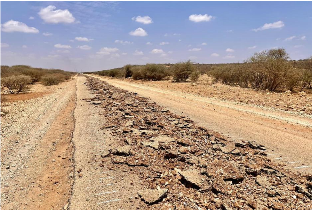
Figure 2 Pavement Scarification
