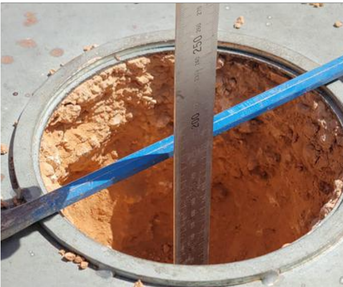
Photo 1: Quality Control Team conducting FDT
