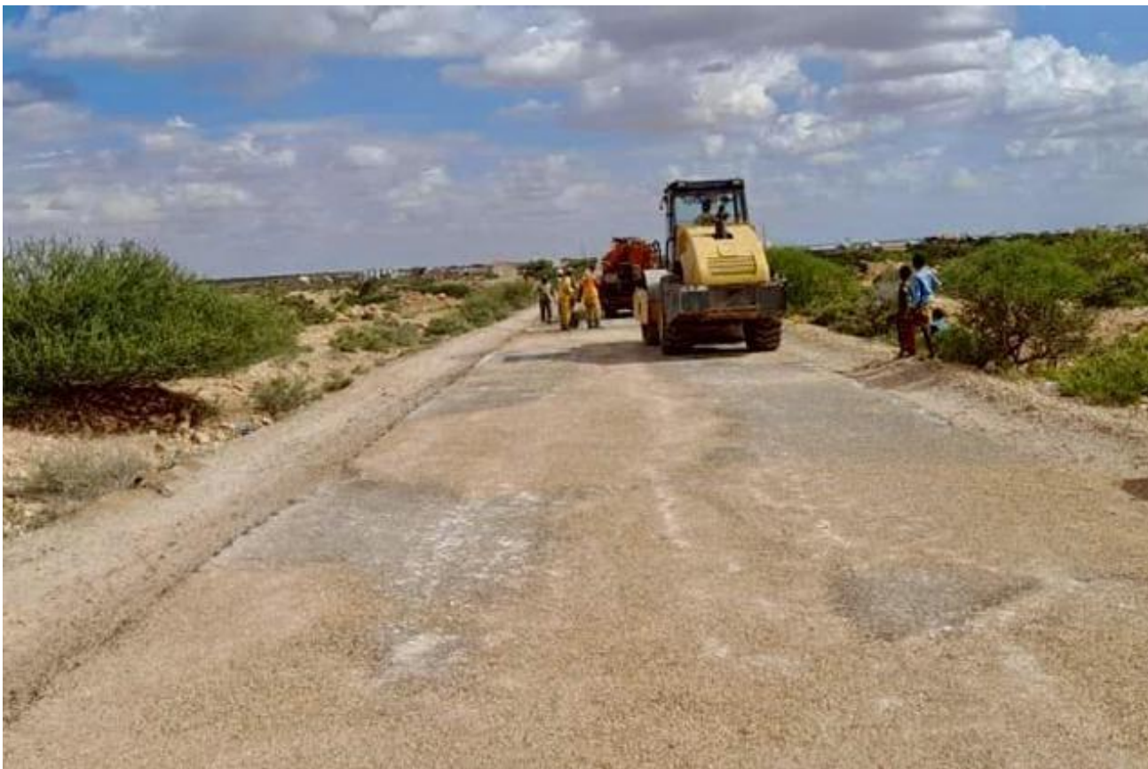
Figure 7 Pothole Maintenance
