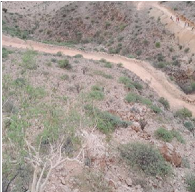
Photo 1: The view of the road
