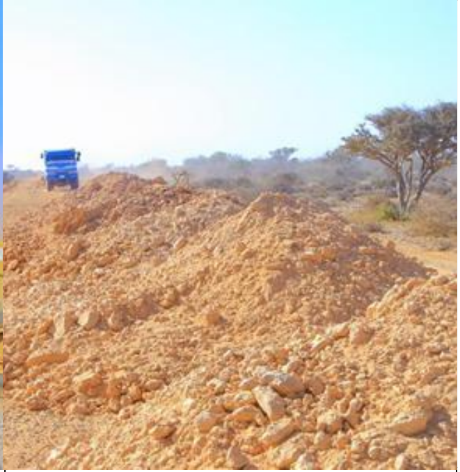
Photo 2: Laying the Sub-base material.
