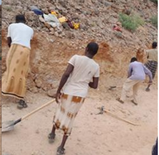
Photo 4:- Ongoing Rock Breaking Process
