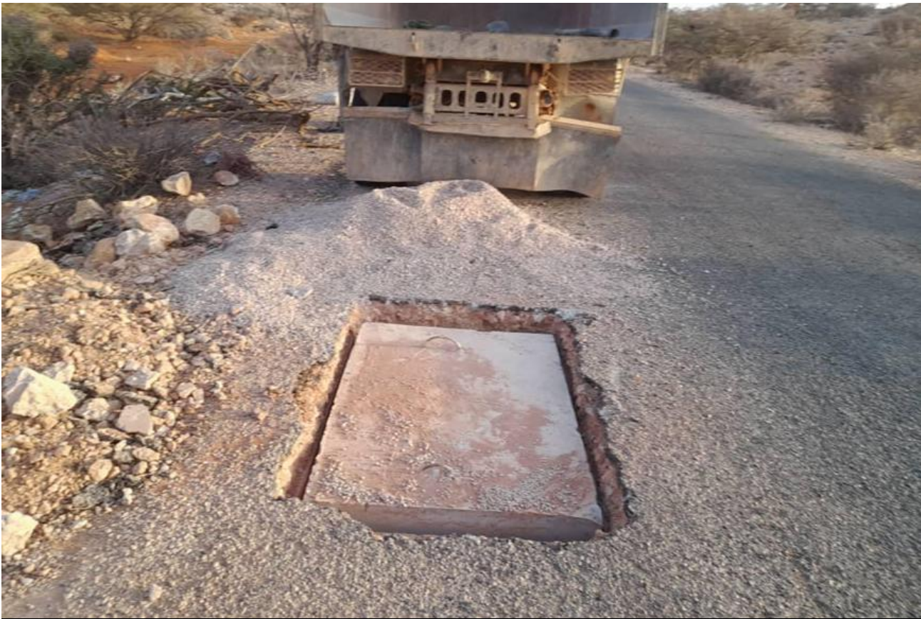
Figure 1 Tuulo - Ooman Culvert rehabilitation
