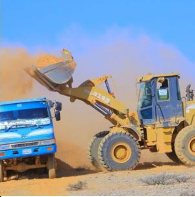
Photo.1: Loading the sub-base material
