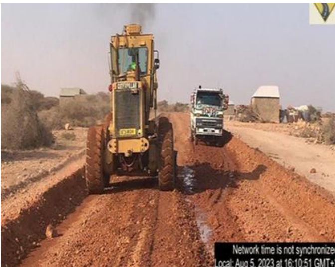
Photo1: levelling and watering the sub-base
