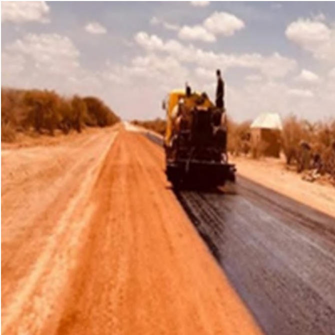
Photo 1: Bitumen Spraying with MC30
