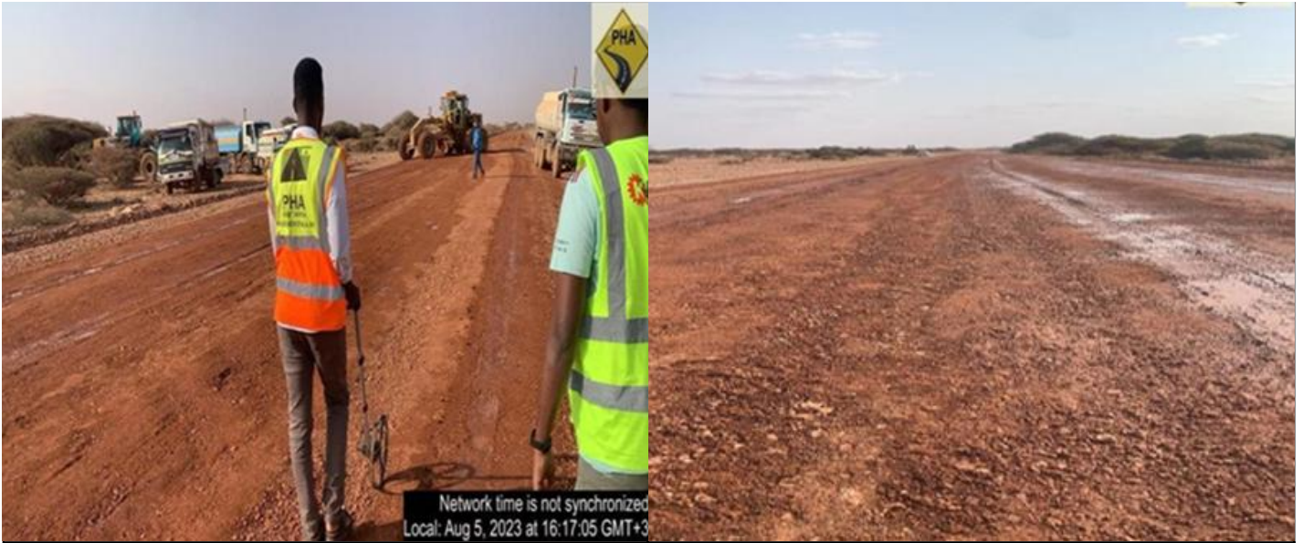
Photo 3: wheel metering for checking the length.
