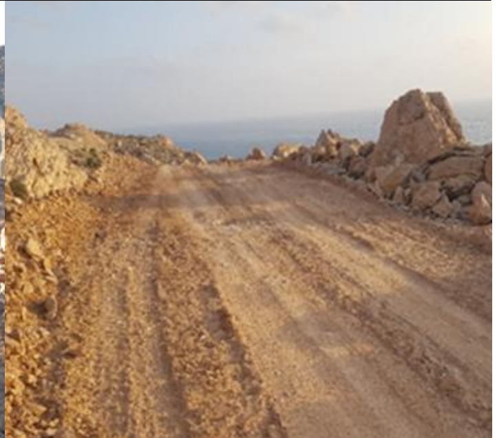
Photo 2: Compacting and levelling.
