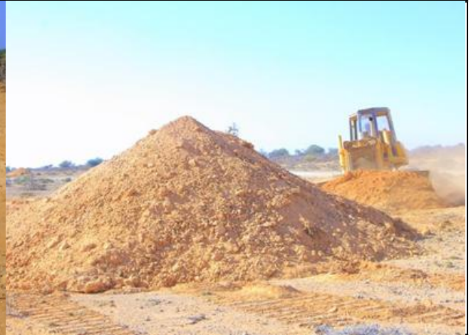
Photo 4: grading and levelling the sub-base material.
