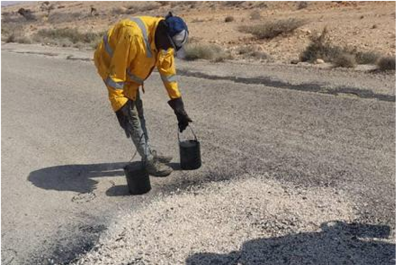
Figure 6: Pothole Maintenances.
