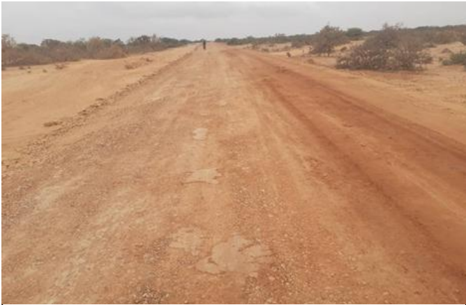
Photo 3: During the Construction process
