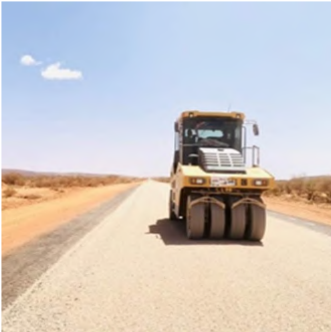
Photo 3: Road Compaction
