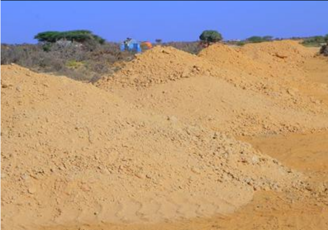
Photo 3: Laying the sub-base material.
