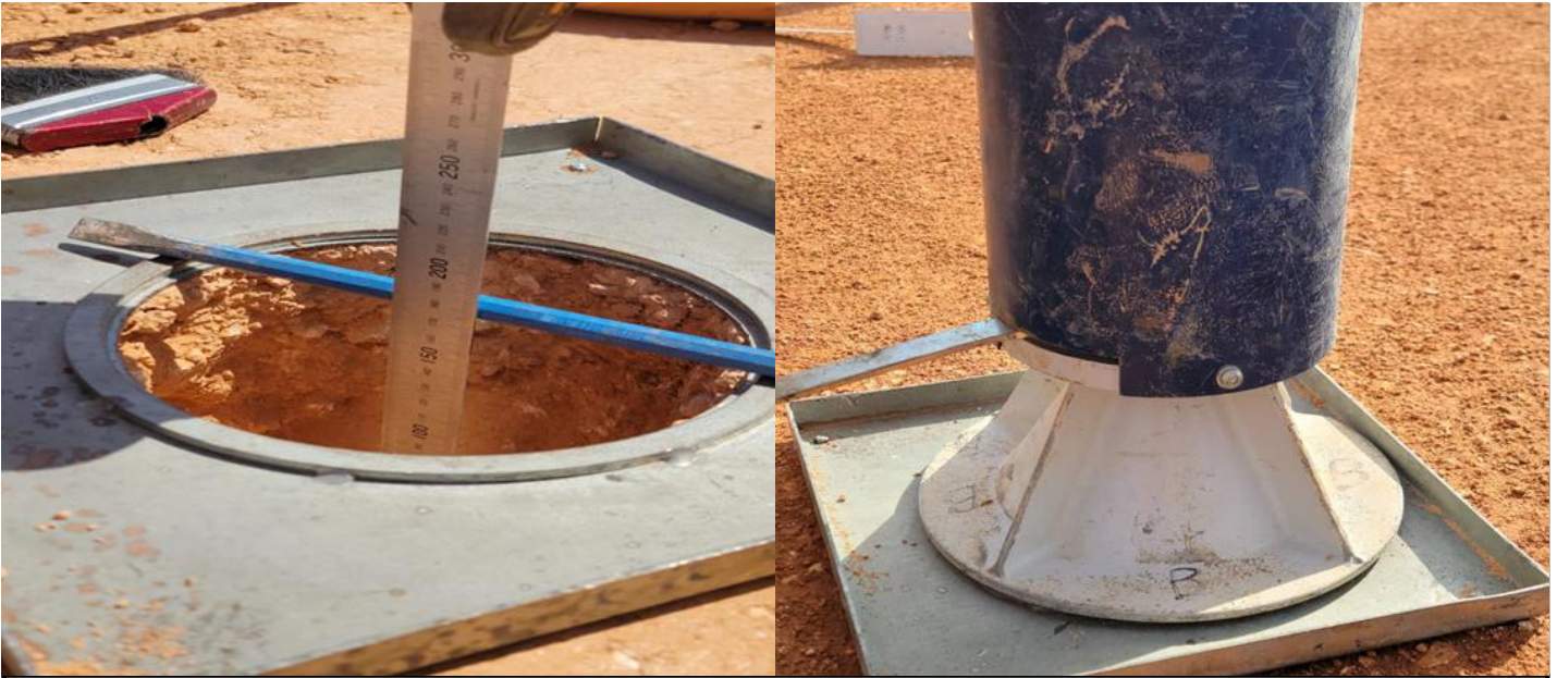
Sand replacement test
