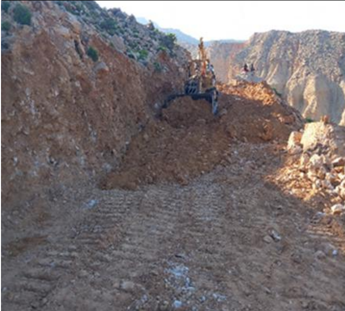
Photo 1: Cutting and Widening process.
