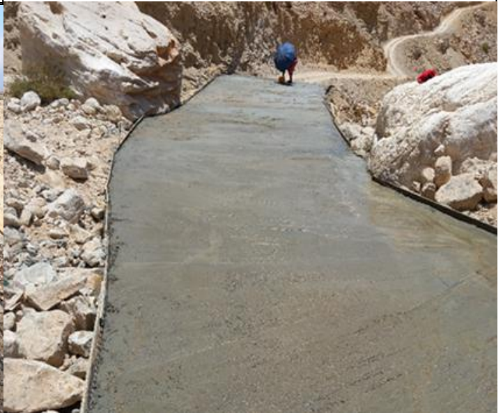
Photo 4: Concrete curing.
