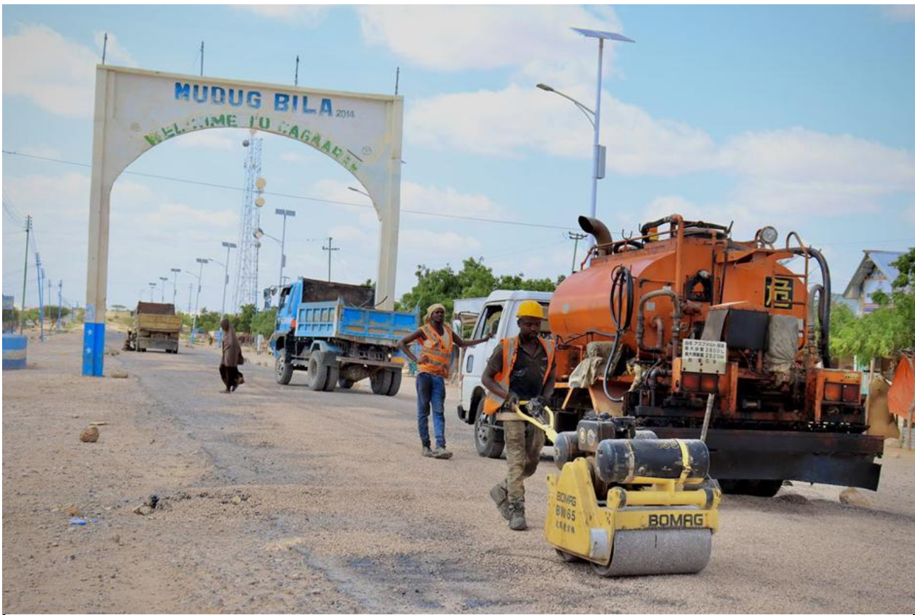
Figure 3: The rehabilitation and maintenance of potholes
