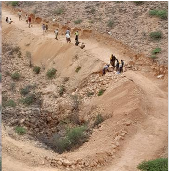
Photo2: The Construction of retaining wall
