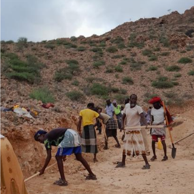
Photo 3: Ongoing Rock Breaking Process
