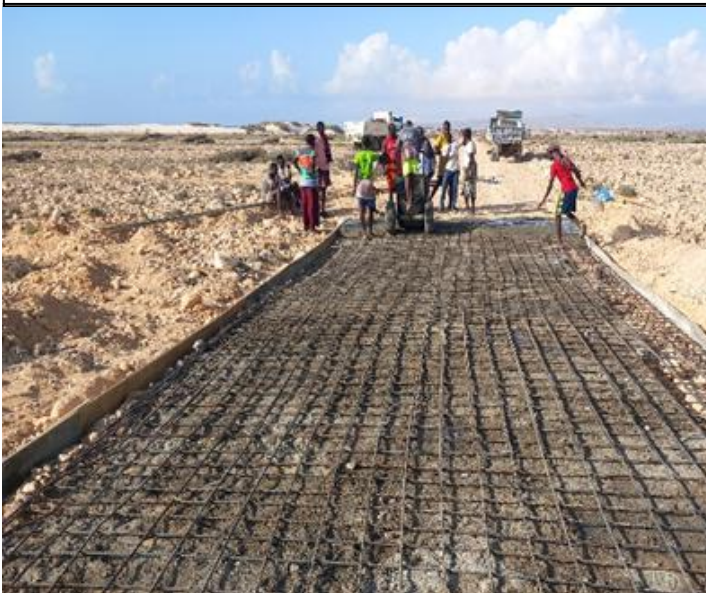
Photo 3: Placing Reinforcement for Drift Structures.
