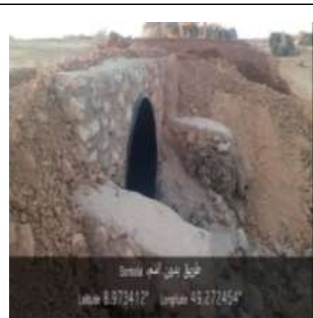
Lat8.973412 Long 49.272454 Photo 52- showing Culvert outlet
