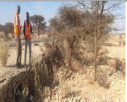
Lat 9.590487 Long 49.152295 Photo 60- showing Culvert outlet
