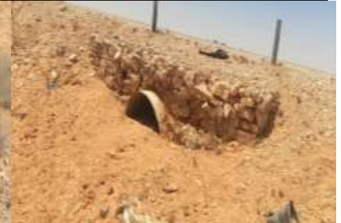
Lat 8.485133 o Long 48.720127 o Photo 9- showing Culvert inlet
