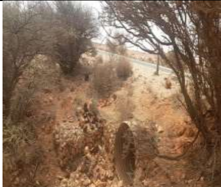
Lat 9.094832 Long 49.210784 Photo 57- showing Culvert outlet
