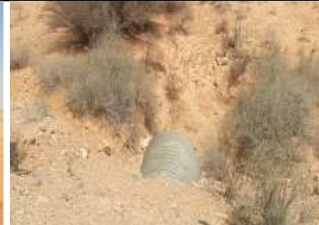
Lat8.475366 Long 48.636227 Photo 6- showing Culvert inlet
