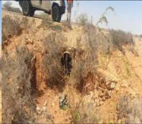
Lat 8.495044 Long 48.757774 Photo 2- showing Culvert outlet
