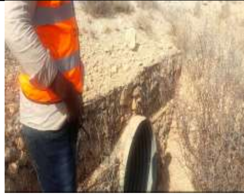
Lat 8.578163 Long 49.045473 Photo 36- showing Culvert outlet
