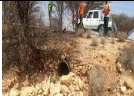
Lat 9.255913 Long 49.106614 Photo 64- showing Culvert outlet
