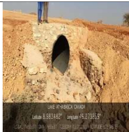
Lat8.983482 Long 49.273859 Photo 52- showing Culvert outlet
