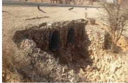
Lat 9.590488 Long 49.152177 Photo 61- showing Culvert outlet
