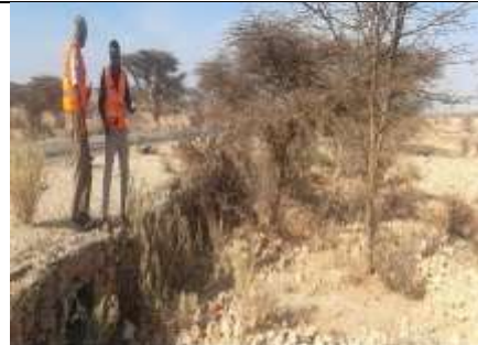
Lat 9.590487 Long 49.152295 Photo 65- showing Culvert outlet
