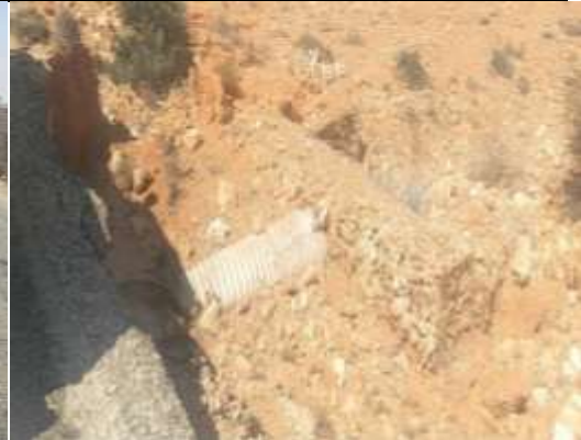
Lat 8.769945 Long 49.336997 Photo 39- showing Culvert outlet
