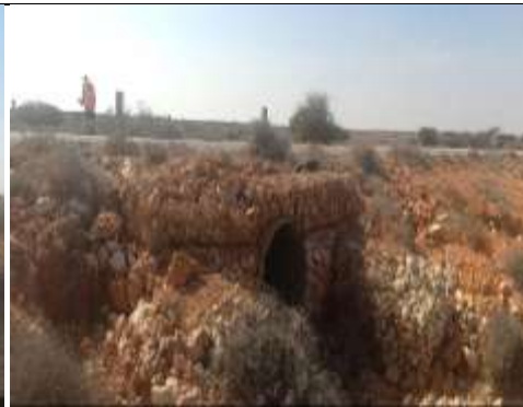
Lat 8.769945 Long 49.336997 Photo 36- showing Culvert outlet
