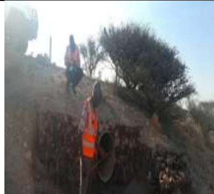
Lat 8.965603 Long 49.274039 Photo 53- showing Culvert outlet
