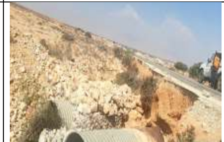
Lat 10.497692 Long 49.074262 Photo 72- showing Culvert outlet
