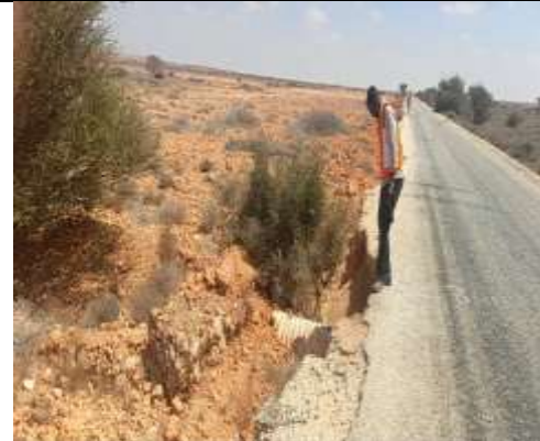
Lat 8.769945 Long 49.336997 Photo 36- showing Culvert outlet
