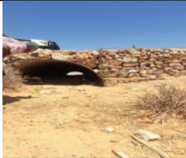
Lat 8.475626 Long 48.609832 Photo 4- showing Culvert inlet
