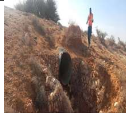
Lat8.930869 Long 49.270730 Photo 52- showing Culvert outlet
