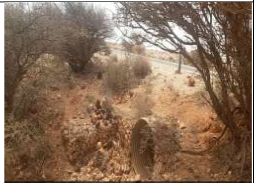
Lat 9.094832 Long 49.210784 Photo 39- showing Culvert outlet
