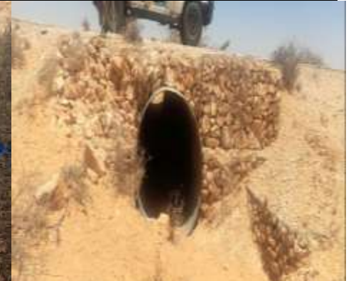
Lat 8.476588 Long 48.645032 Photo 7- showing Culvert inlet
