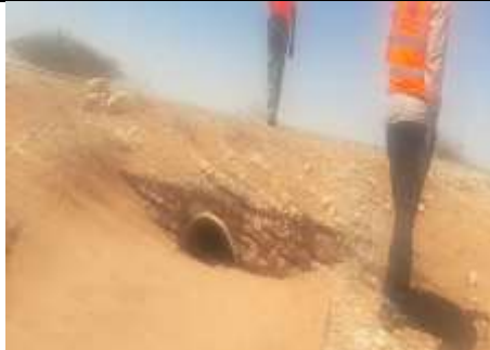
Lat8.488484 Long 48.732844 Photo 5- showing Culvert inlet
