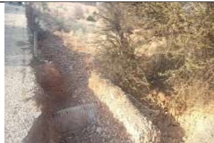
Lat 9.658915 Long 49.174339 Photo 68- showing Culvert outlet
