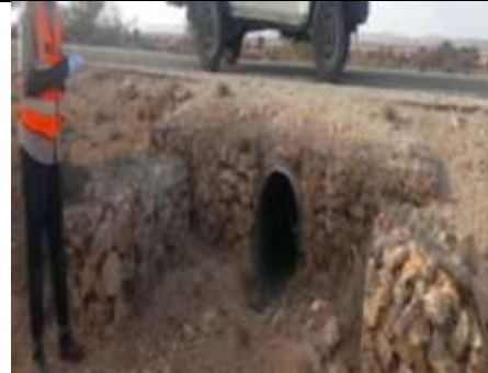
Lat 8.588438 Long 49.106712 Photo 36- showing Culvert outlet
