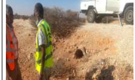
Lat 9.750158 Long 49.195473 Photo 70- showing Culvert outlet
