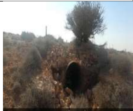
Lat 8.769945 Long 49.336997 Photo 36- showing Culvert outlet
