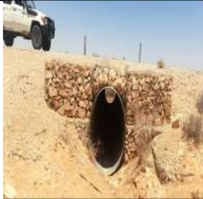
Lat 8.476201 Long 48.642633 Photo 1- showing Culvert inlet
