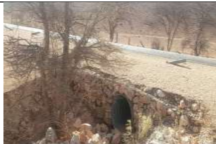
Lat 9.590824 Long 49.152363 Photo 67- showing Culvert outlet
