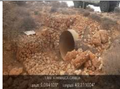
Lat 9.114340 Long 49.199204 Photo 59- showing Culvert outlet
