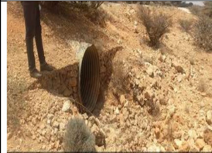
Lat 9.198716 Long 49.133525 Photo 66- showing Culvert outlet
